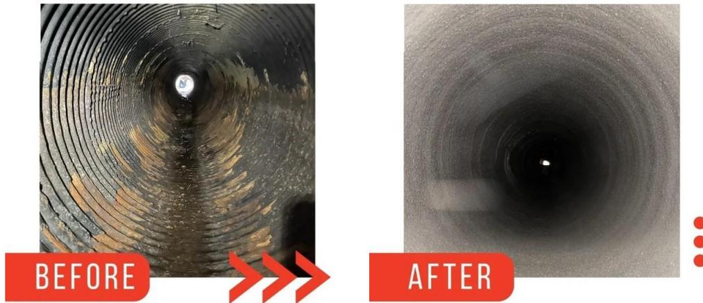
Figure 4. On the left, the raw metal pipeline; on the right, the shotcrete lined pipeline after restoration.
