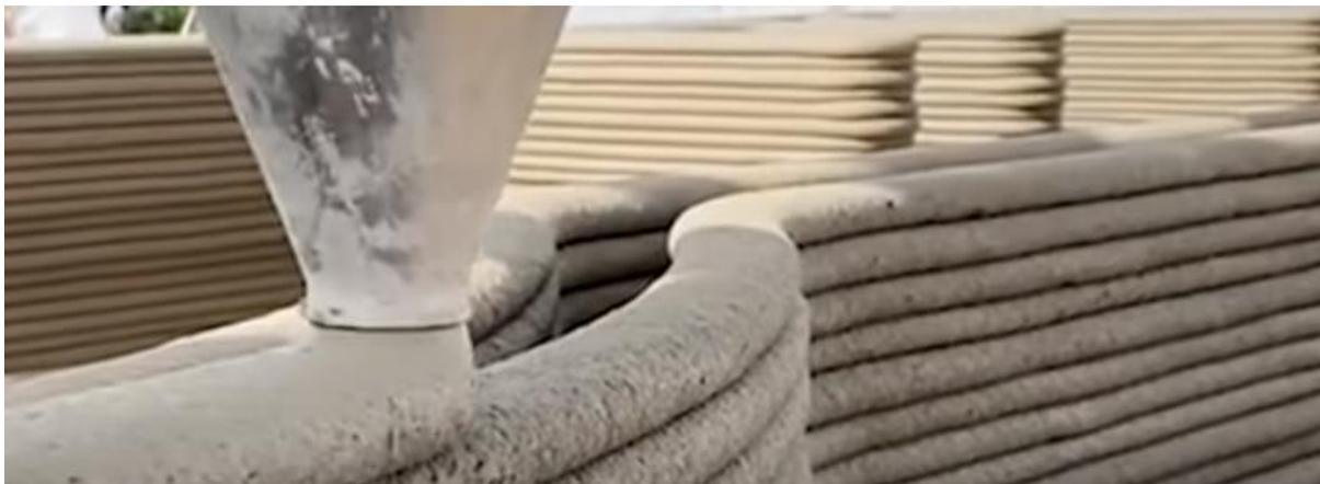
Figure 3. 3D concrete printing trial
